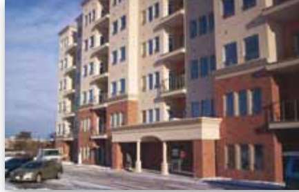
Nottingham Gate Oakville Ontario, Kanada
